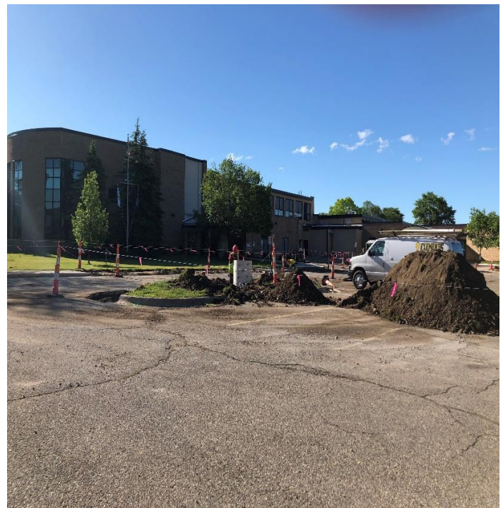
Excavation for Light Pole Bases
