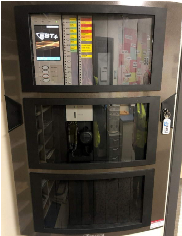
New Fire Alarm Panel (typical for all updated systems)
